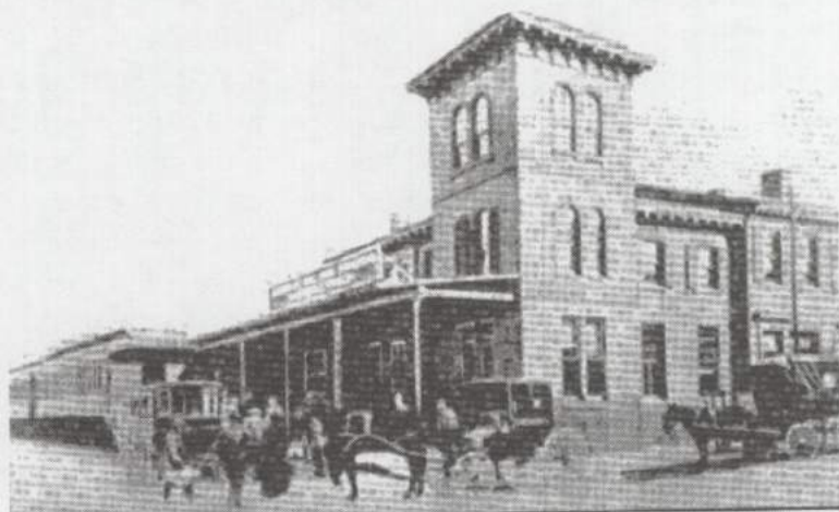
The B&O station at South Market and All Saints streets had many famous visitors before it was closed and the tracks removed. It is now home to the Frederick Community Action Agency.
