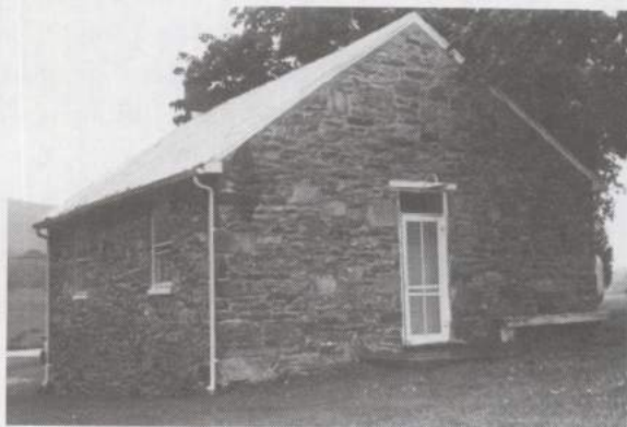
Native stone was used in the construction of Bethel School (construction date unknown).
