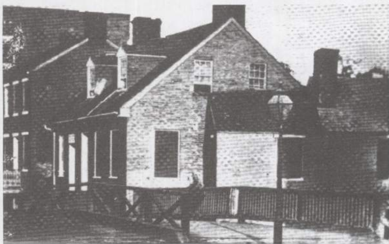
A replica of Barbara Fritchie's home replaced the original, which was badly damaged during the flood of 1868.
