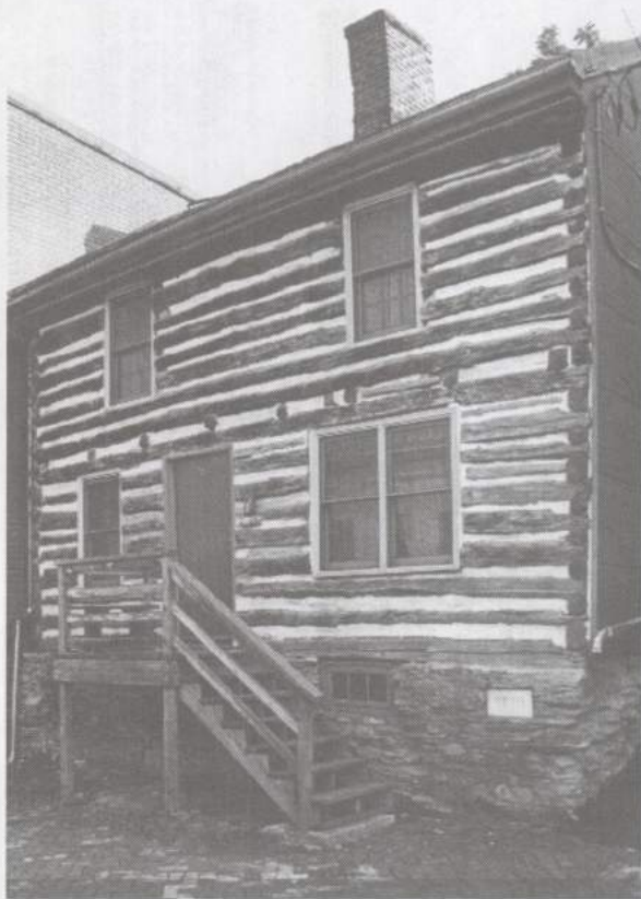
This log house, dated 1770, is still standing and being used as a residence. It is typical of early Frederick architecture.
