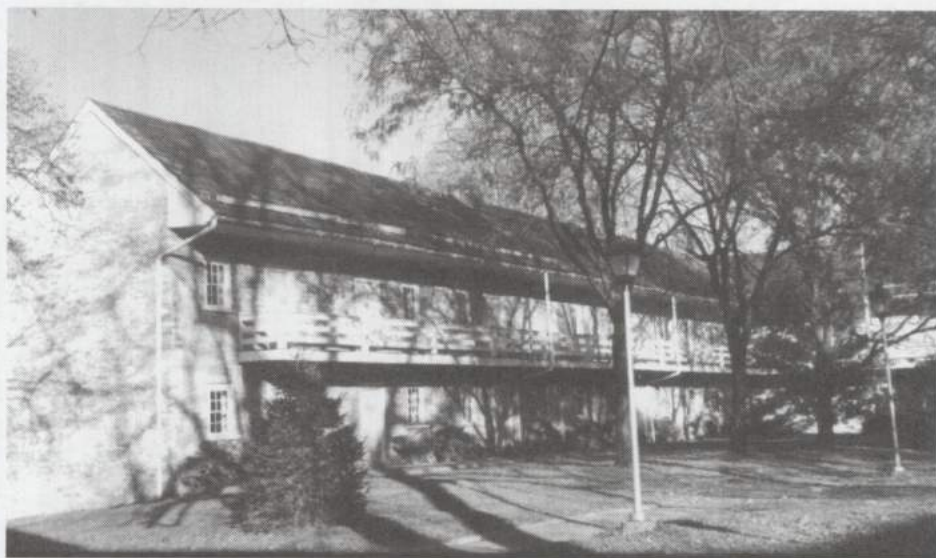
Among several uses of these barracks through the years was the housing of Hessian soldiers captured during the battle of Yorktown, in the Revolutionary War. One of two buildings is standing today, and is used as a museum.
