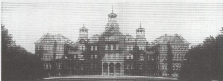
This old building housed the Maryland School for the Deaf on South Market Street for almost 100 years. Jacob Engelbrecht noted its construction in his Diary.
