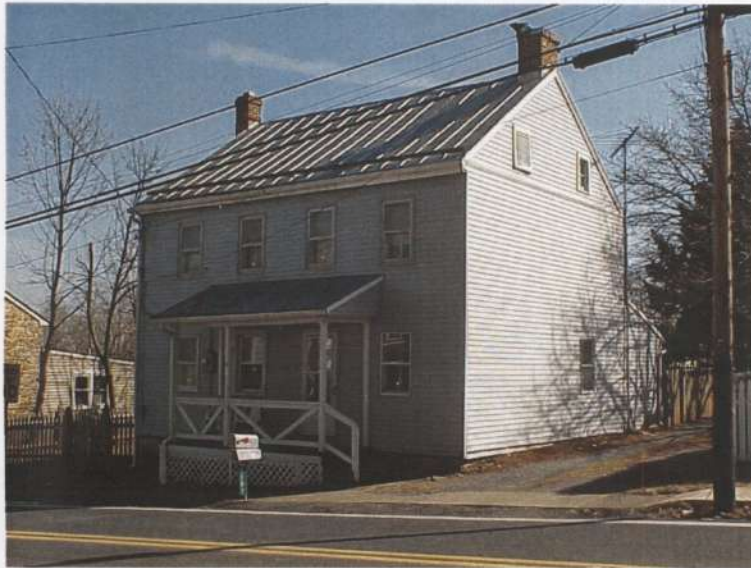
This house is log under the wood siding.
