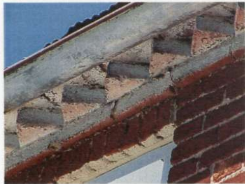
Three brick courses under the roof are set on the diagonal.
