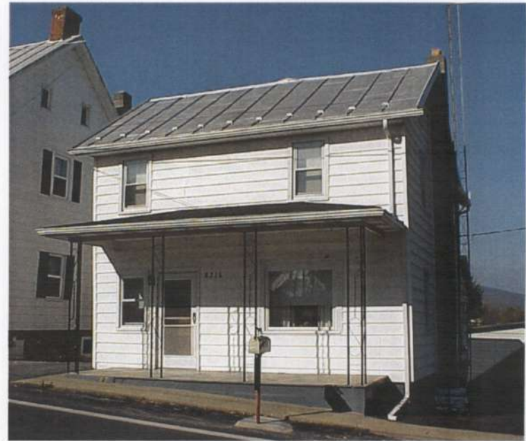
This house was probably built in 1786 by Peter Guenther. It is log under the siding.
