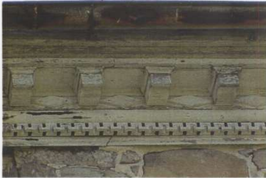
A portion of the south soffit.
