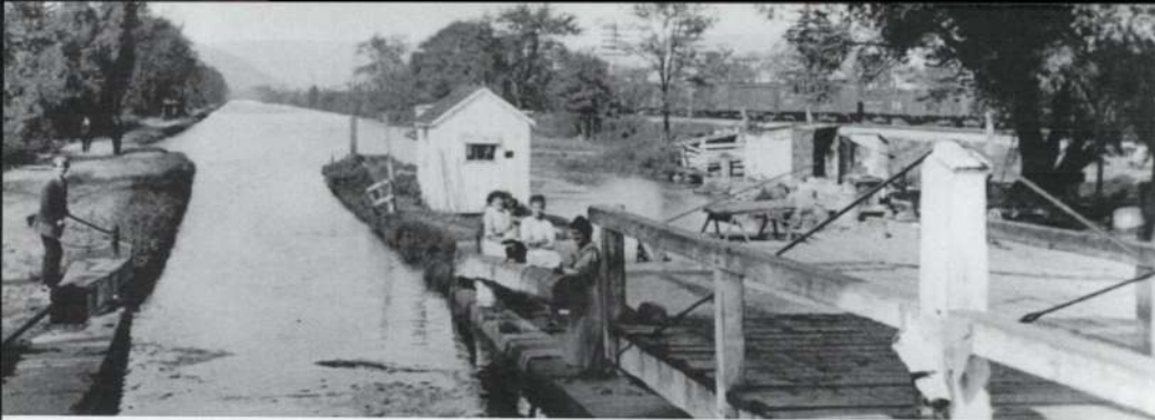
◆ Although later eclipsed by the railroad, the C&O Canal was a major route for trade in the emergent American republic. This is Lock 30 near Brunswick, Maryland.
