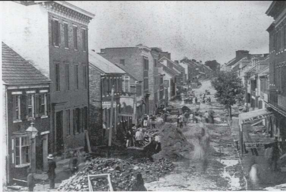
◆ Frederick's industrial district along Carroll Creek was prone to flooding through much of the city's history prior to flood control efforts in the late 1970s. This image shows the flood damage on West Patrick Street during an 1868 flood.
