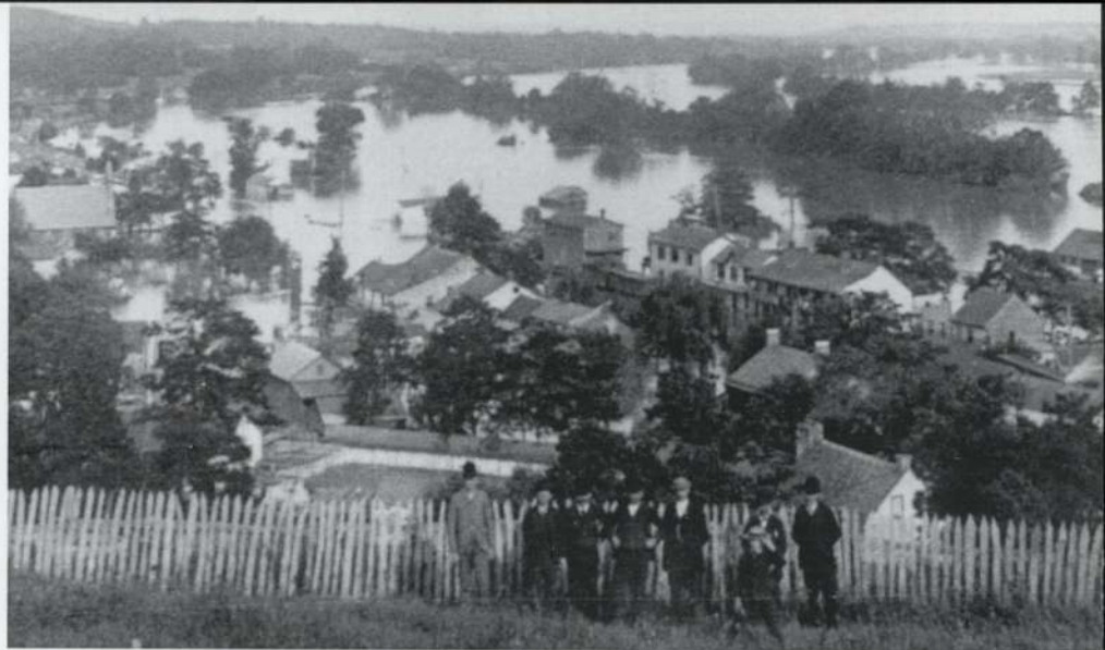
❖ Point of Rocks flooded by the Potomac River in 1889, in which much of the town, including the railroad tracks, was under water.
