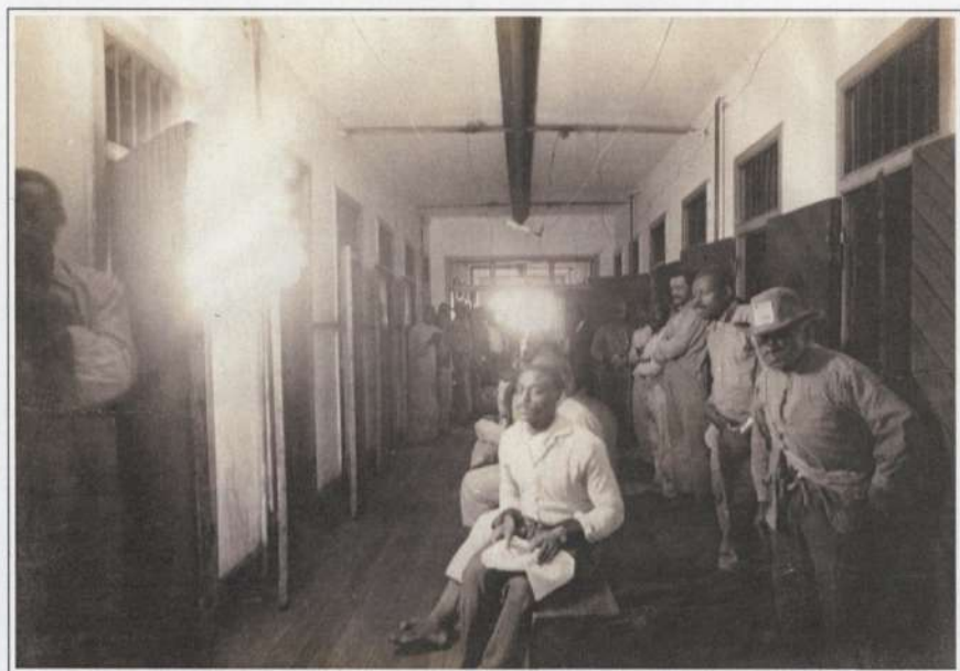
View of the male African-American ward in the Old House, circa 1909. A photograph taken for the Lunacy Commission Report. The photograph was taken prior to improvements that were made in 1910. Collection of the Maryland State Archives.
