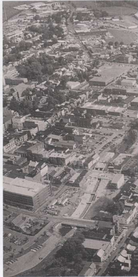
Aerial view of the middle section of the Carroll Creek flood control project.
