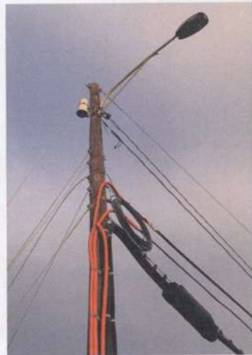
Ugly overhead powerlines disappeared when they were buried on South Market
