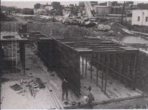
Massive underground culverts divert raging storm waters to prevent flooding.
