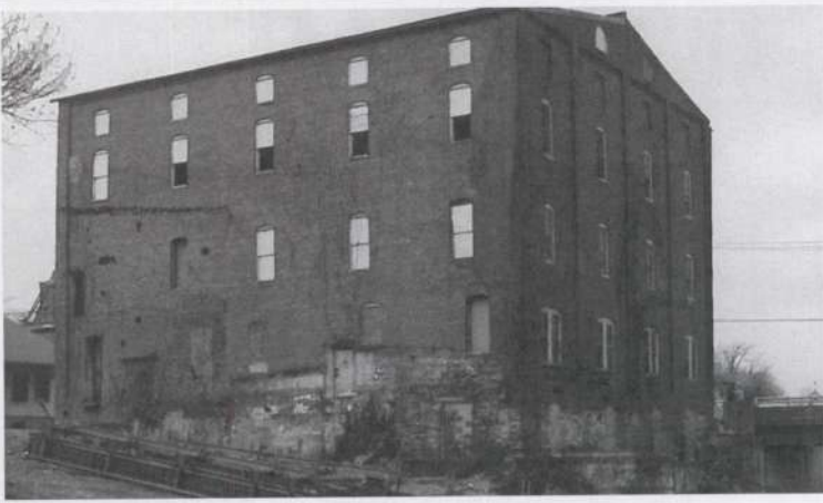
The former Mountain City Mill was transformed into the Delaplaine Arts Center.
